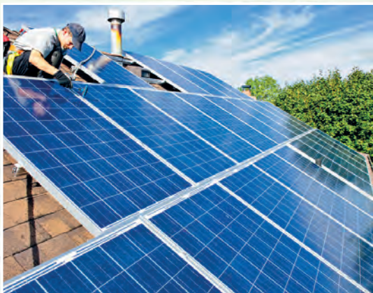
Solar Panels for Free electricity
